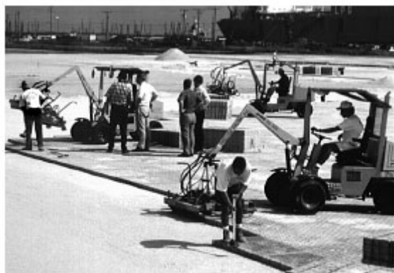
Figure 9. Mechanical installation equipment places concrete pavers rapidly.
